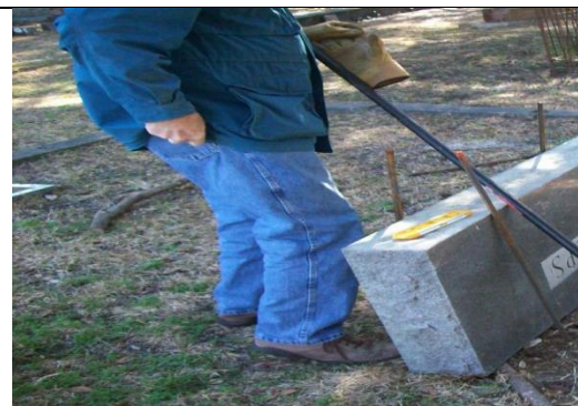
Phelps stone upside down while the base is having pebbles pushed under it to make it level.
