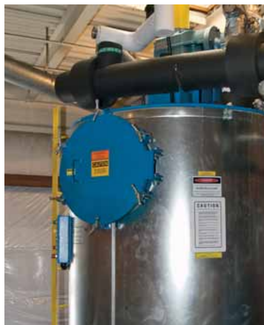
Used ink is piped to this holding container where it is processed for recycling. Some 3,500 gallons of alcohol “sludge” is sold every three weeks for firing brick kilns.
